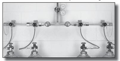
The 633 Series Duplex supports two banks of high pressure cylinders for applications where continuous gas supply is not required. A heavy-duty valve manually controls the bank priority, and line or station regulators should be installed at the point of use to ensure constant delivery pressure. Use of Acetylene requires flashback arrestor on pigtails.
