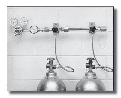
The 631 Series Simplex combines a modular manifold system with the extra heavy-duty 6700 Series regulator. Line or station regulators should be installed at the point of use to ensure constant delivery pressure. Use of Acetylene requires flashback arrestor on pigtails.
